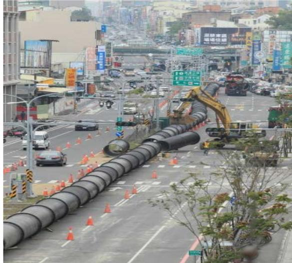
Fig.3 1,350 mm emergency temporary transmission pipe on the ground
